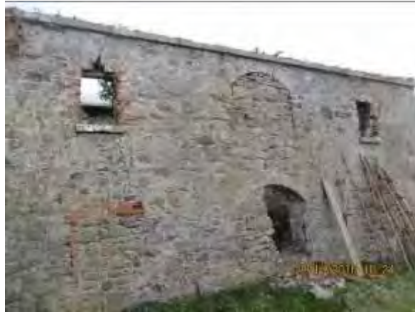
Photograph 2 View of exterior wall of subject buildings from site.
