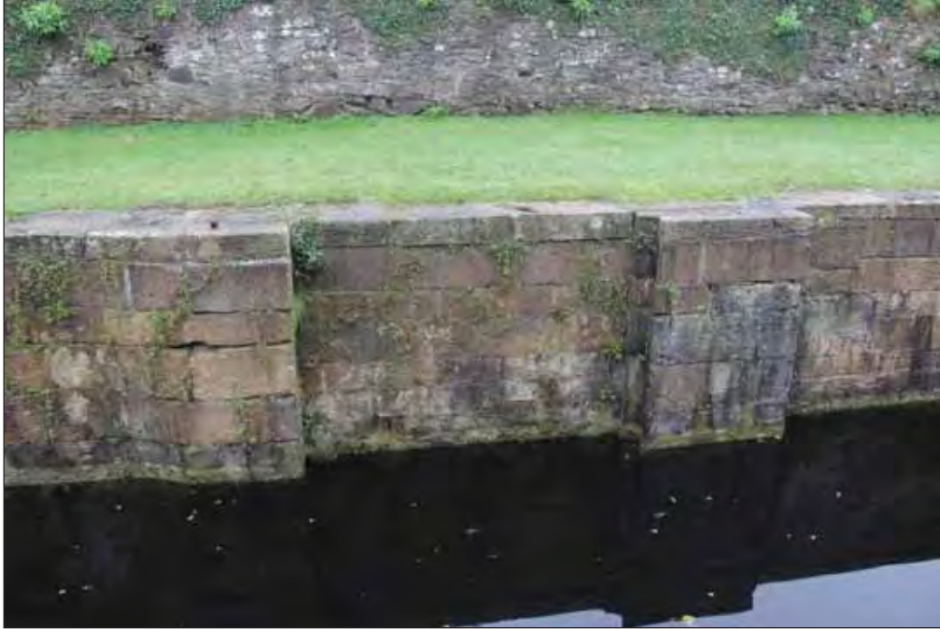
Photo 6 - The Old Lock Bridge
