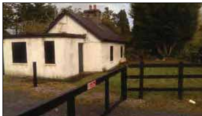
Photo 40 – View of Deey Bridge Lockhouse from Towpath
