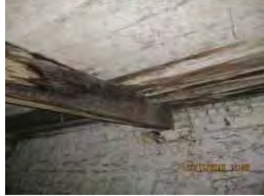
Photograph 2 Joist to First Floor
