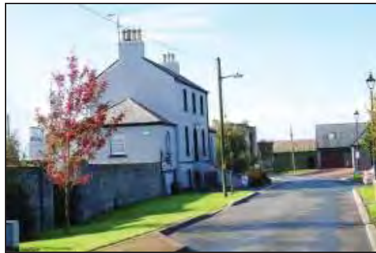
Photo 33 - View along the South Towpath Showing the Former Canal Master's House.
