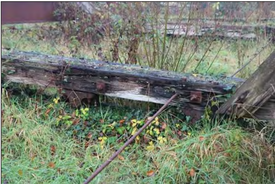
Photo 5 - Main Sliding Beam - Cast Iron Wheel/Runner
