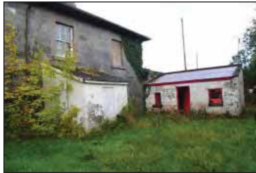
Photo 21 - Rear View of House and Sheds
