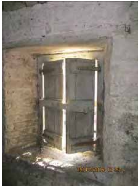
Photograph 7 Internal view of existing window assembly
