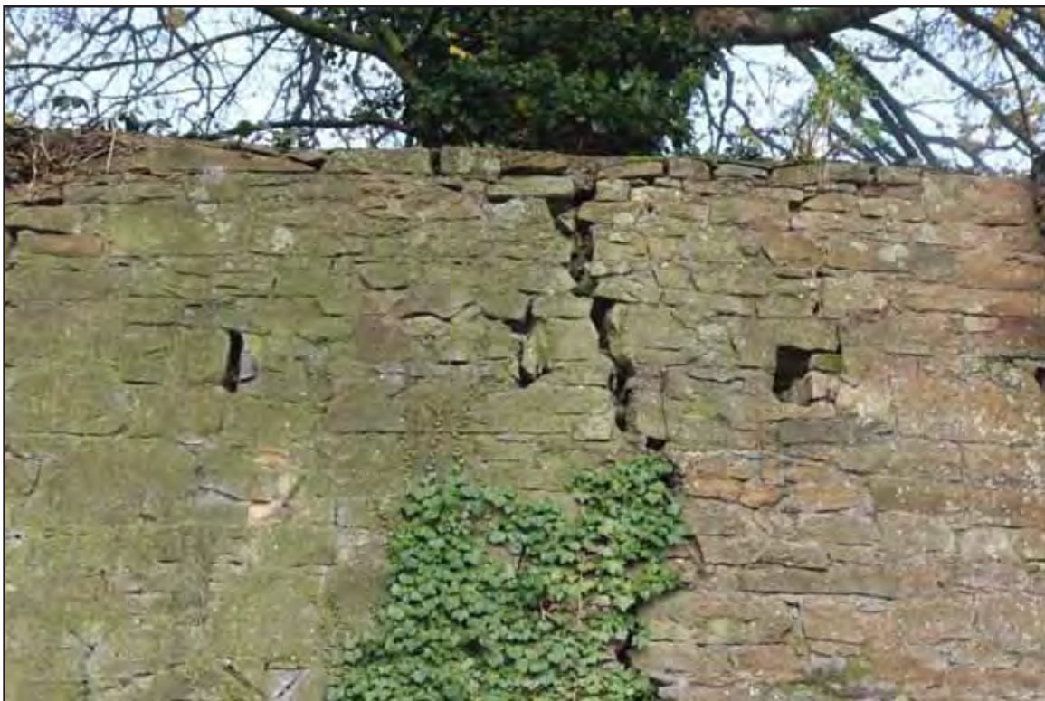
Photo 2 - Section of Cathedral Wall to be Monitored
