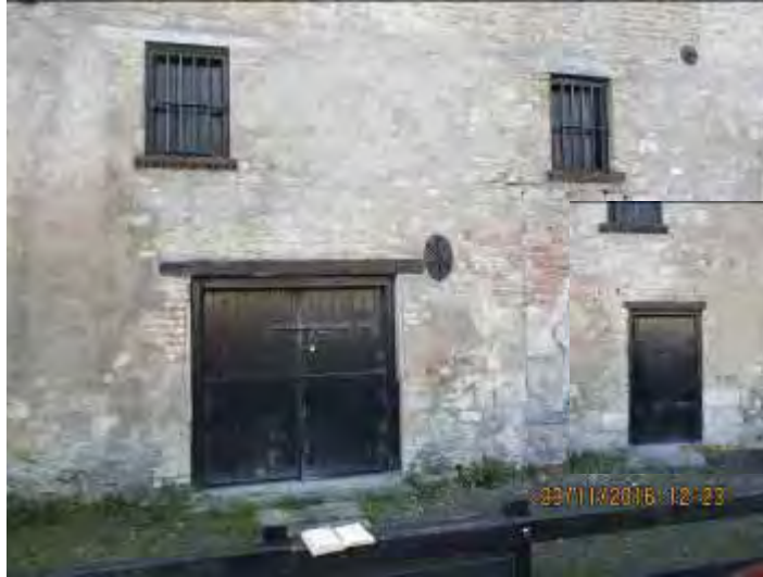
Photograph 8 View of external doors (main and inset)
