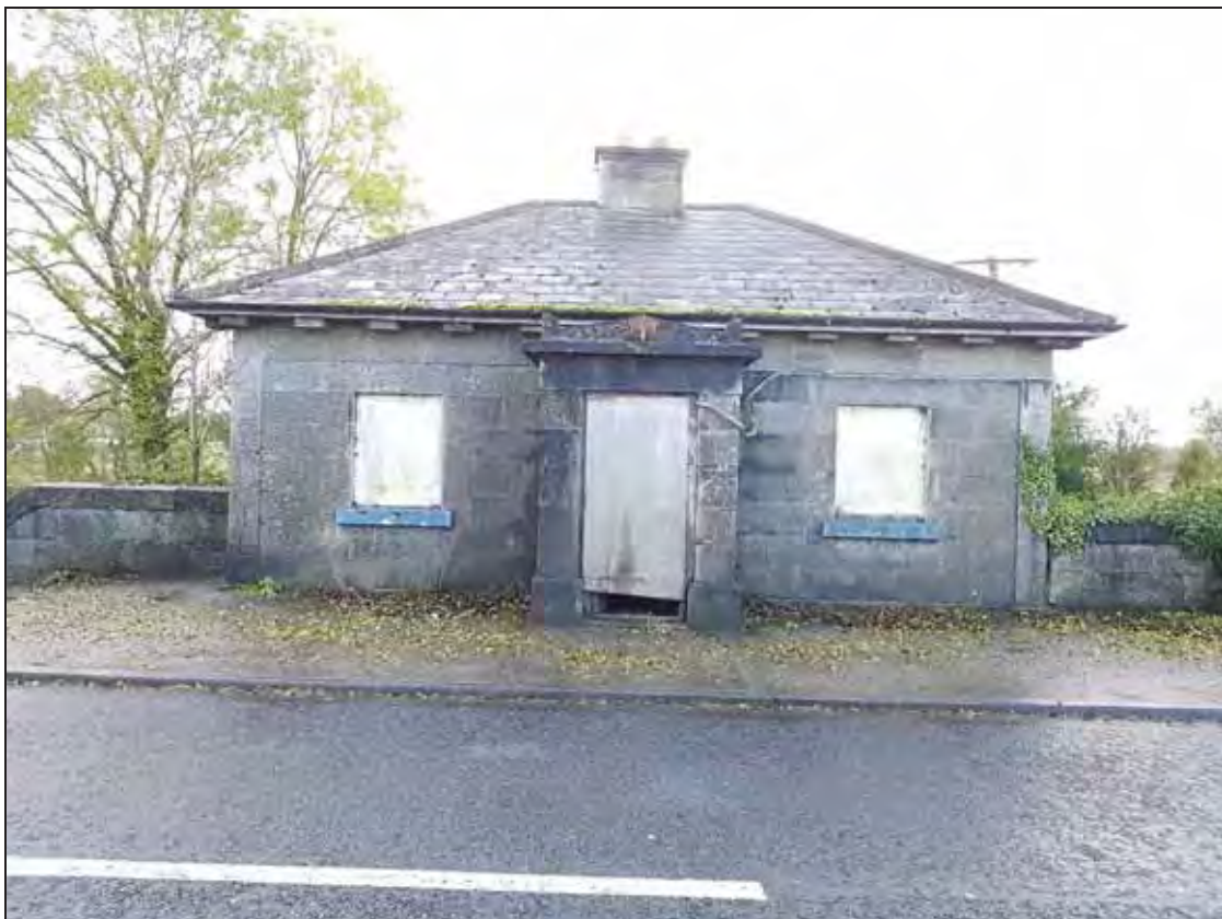
Photo 14 - Bridge Operator's House (Site Visit October 2016)
