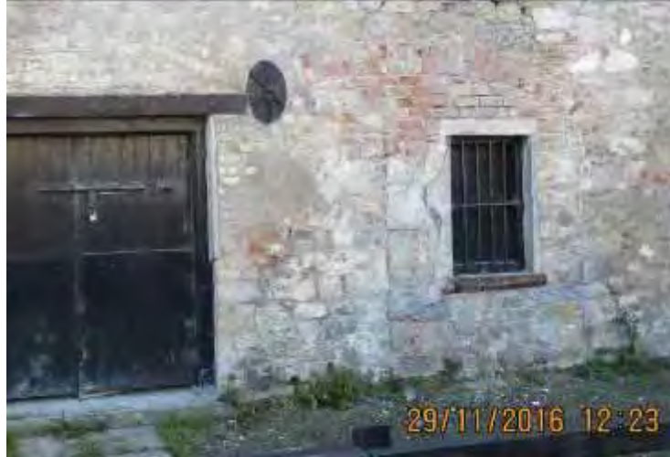
Photograph 4 View of front facade
